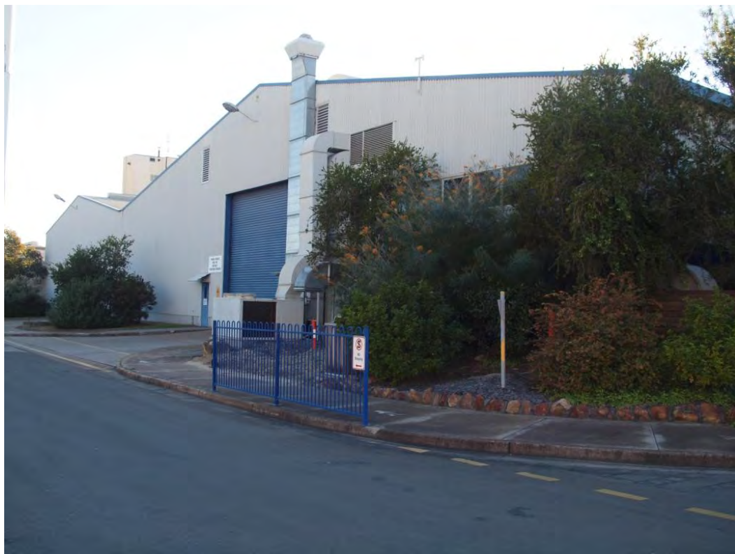
Plate 24 Ancillary buildings – Engineering
