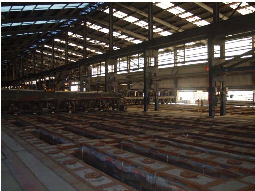
Plate 6 Carbon Plant – interior
