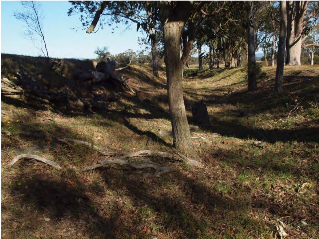
Plate 37 South Maitland Railway cutting deviation - Glen Greta (Glen Main) Colliery subsidence (looking south)
