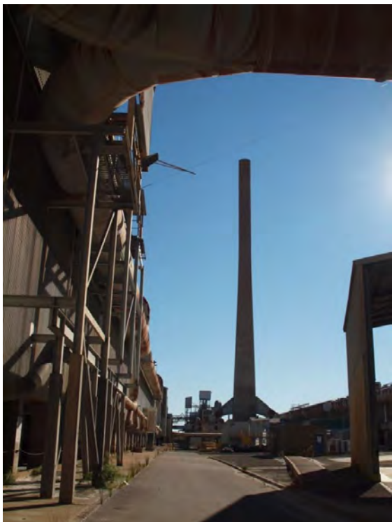
Plate 20 Looking north to chimney
