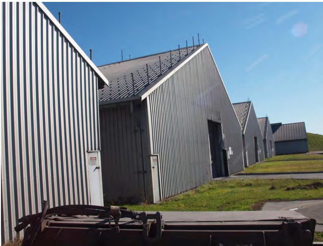
Plate 27 Ancillary building - Potline storage sheds
