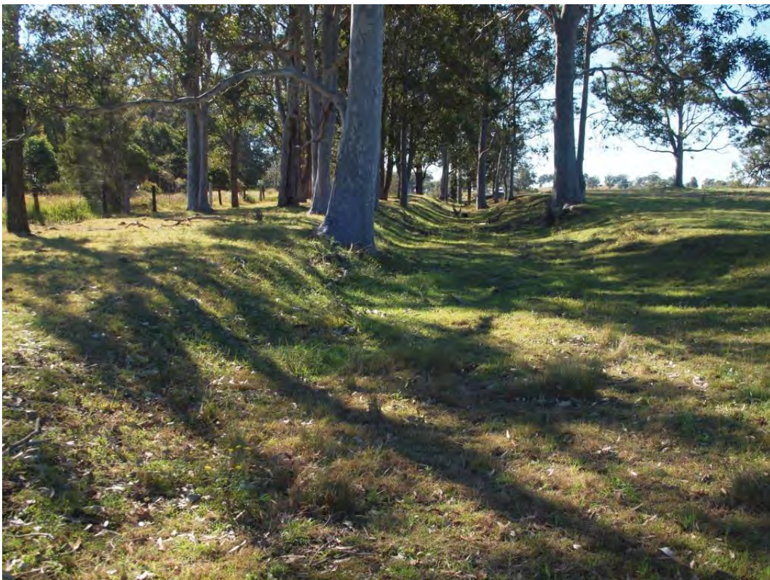
Plate 36 South Maitland Railway cutting deviation - Glen Greta (Glen Main) Colliery subsidence (looking north)
